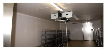
Description: Insulation based polyester panel with aluminum vapor barrier
